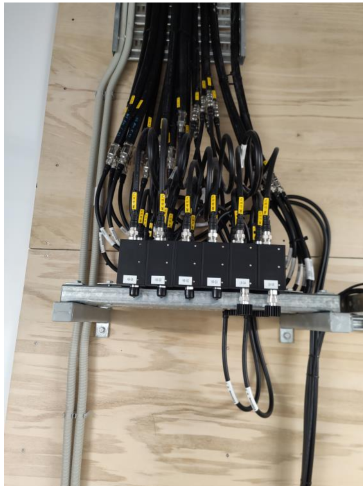
Cell site antenna distribution for a mall
