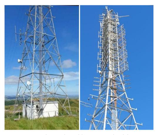
Progress on replacing the Cable Trays on Klondyke Tower The increased width avoids coaxes being stacked on each other
